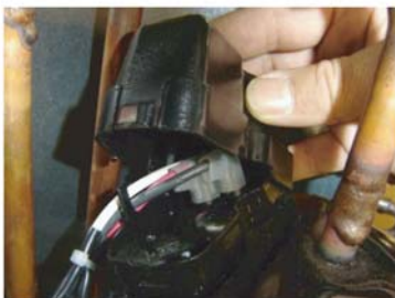
Remove the TERMINAL COVER.
