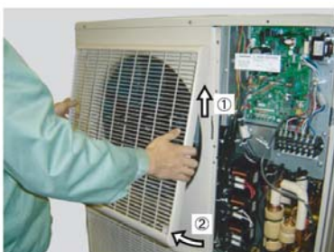
Remove the FAN GUARD by sliding upward.
